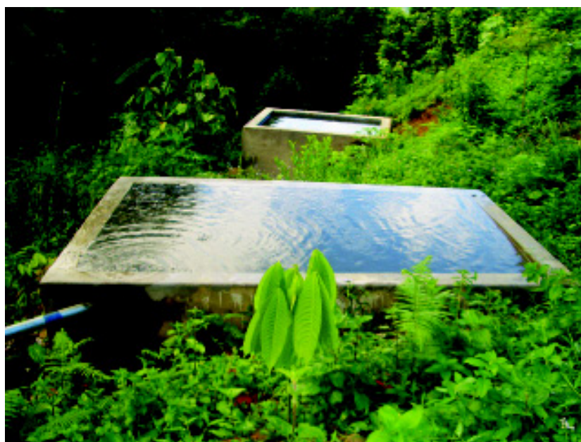
Fig 1. Spring water and base flow harvesting in series of tanks
