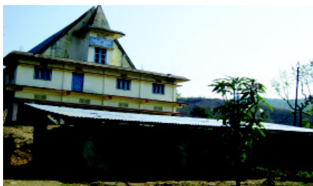
Fig 2. Roof water harvesting from church for multiple use
