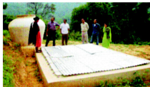
Fig. 2 Jars and ferro-cement lined tanks for intermediate water storage, and is an important element of MUS
