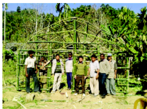
Fig. 1 Construction of low cost poly house at Lida village
