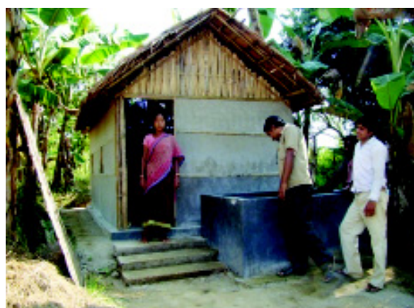
Fig 1. Newly constructed mushroom sheds
